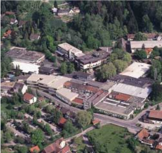
Aerial view Lindau-Rickenbach works
