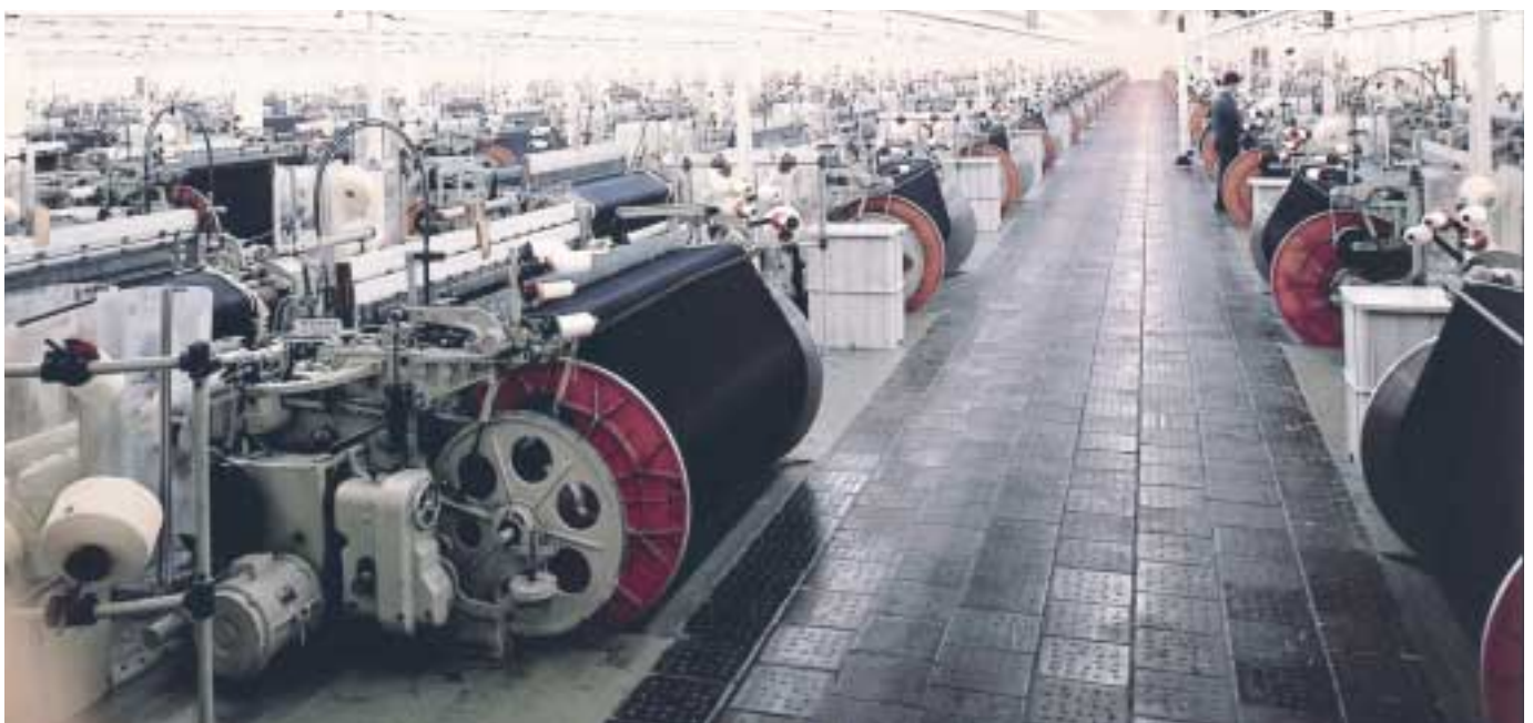
The DORNIER Rapier Weaving Machine installation at the Spanish company Iberica de Confecciones 1976
