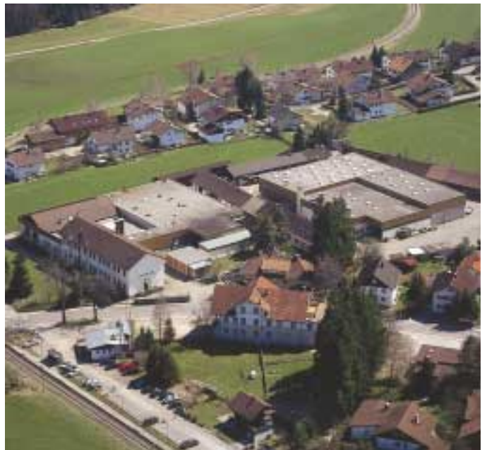
Aerial view Pfronten works
