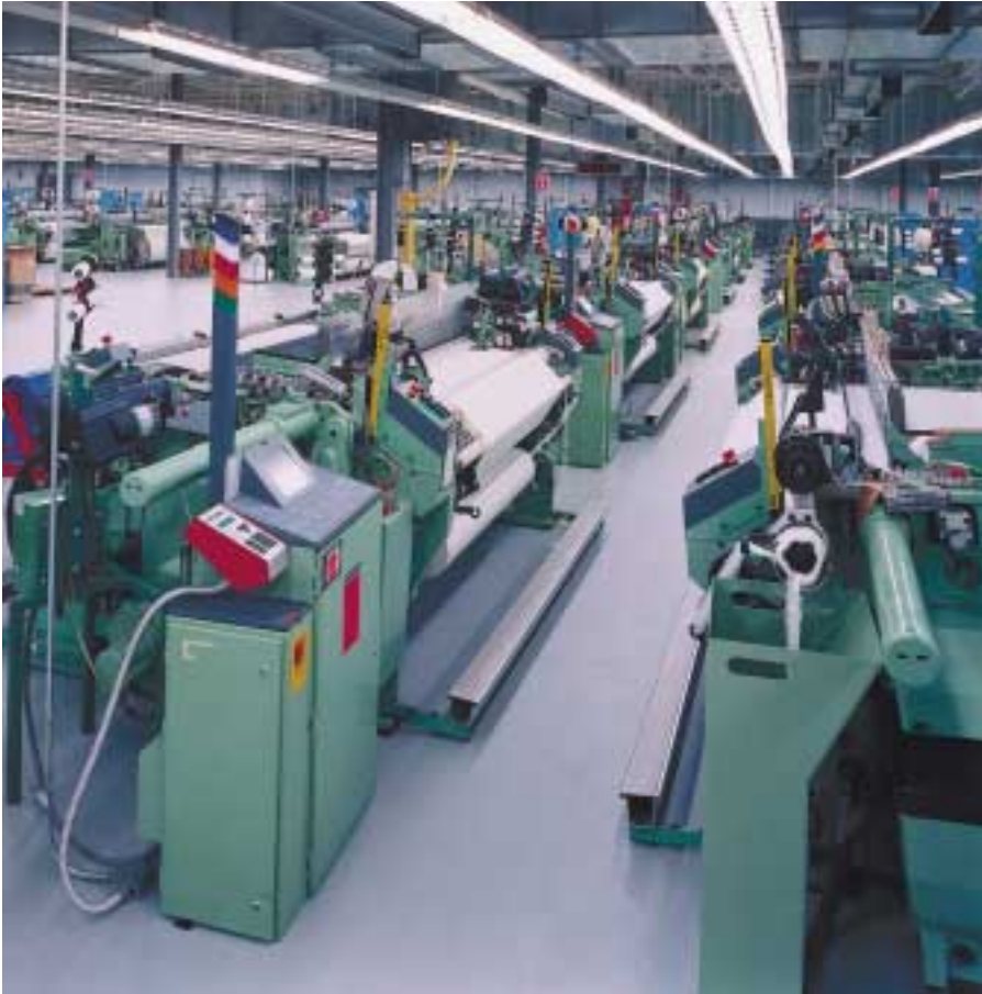
The DORNIER Rapier Weaving Machine installation at Southern Mills
