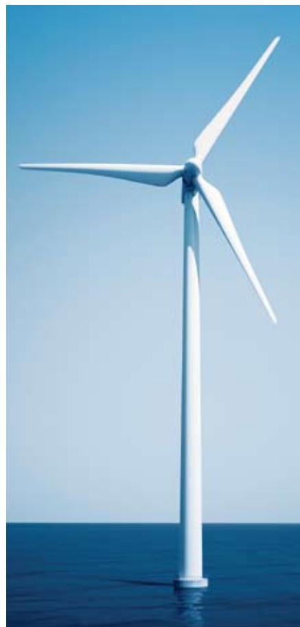
Off-shore wind power unit with GFRP/CFRP material
