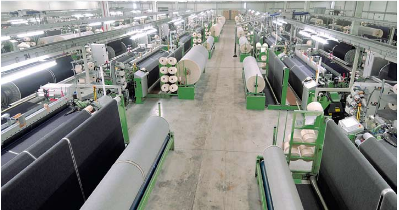
Modern weaving plant in Turkey with DORNIER A1 air-jet weaving machines for denim
