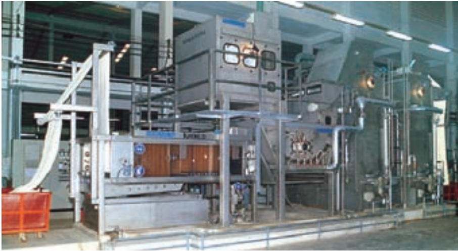
EcoCombine® mercerizing-bleaching plant in Thailand
